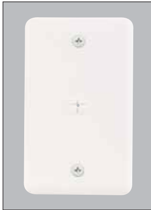
Finished Installation of the A-465
