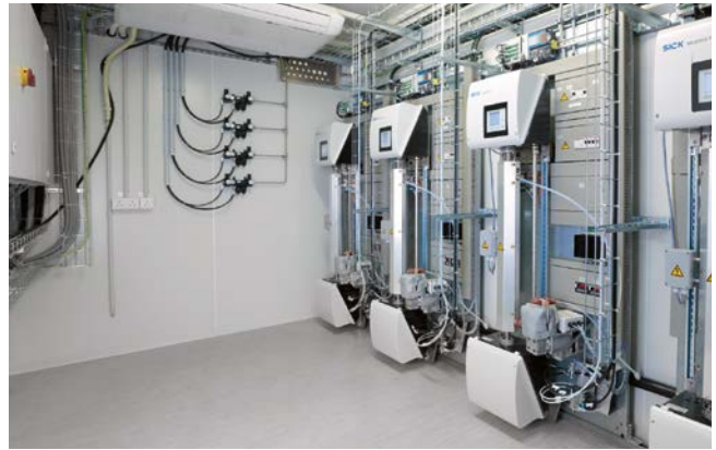
MCS300P Ex Wall housing, can optionally be used in Ex zones 1 and 2 → Page 23
